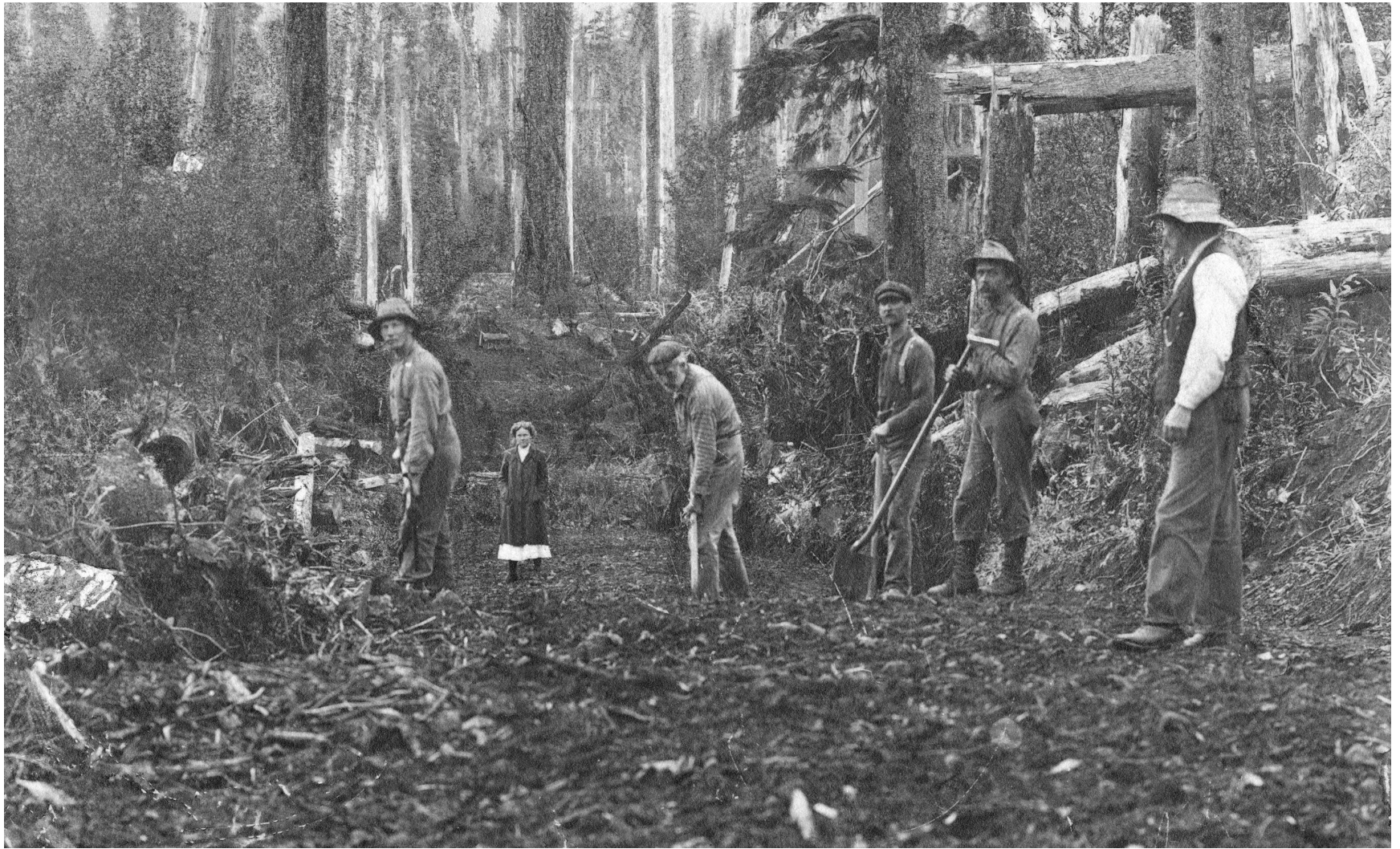
Quatsino settlers building a wagon road between Coal Harbour and Hardy Bay (1909)
