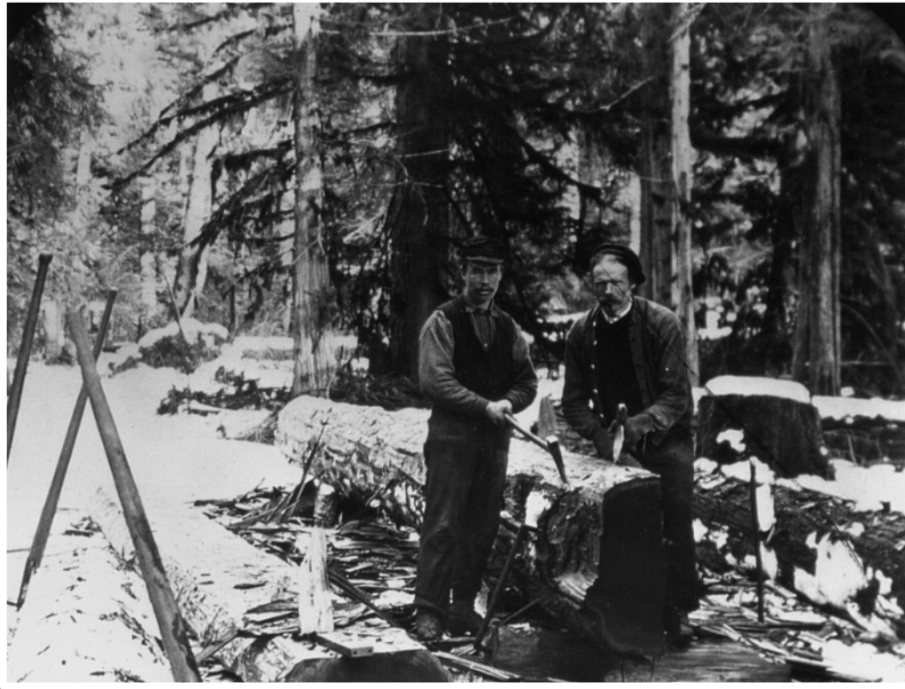
Andrew Svidahl, left, and Mathis Hammer, two of the original Norwegian settlers, squaring timber for construction.
