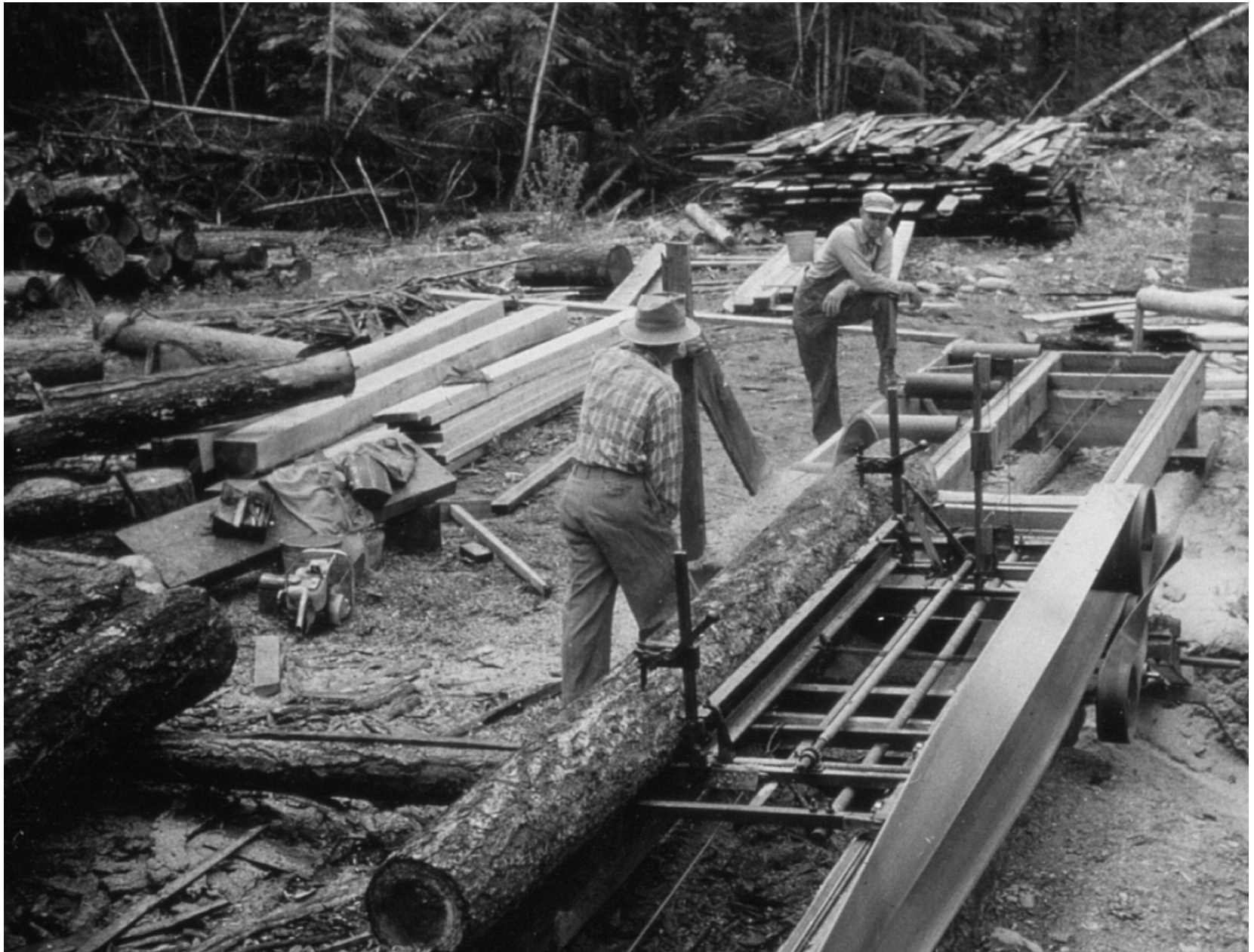
Elmo Wolfe and Bob Boyd hewing timber in the late 1950s for the construction of Argenta Friends School.
