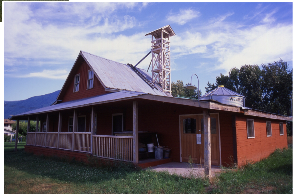
Right: Beautifully restored, but with slightly modernized machinery, this 1915 flour mill still produces modest quantities of flour, bran and animal feed for local health-food and specialty stores.
